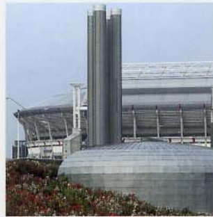
Central heat supply unit, Amsterdam, Netherlands
