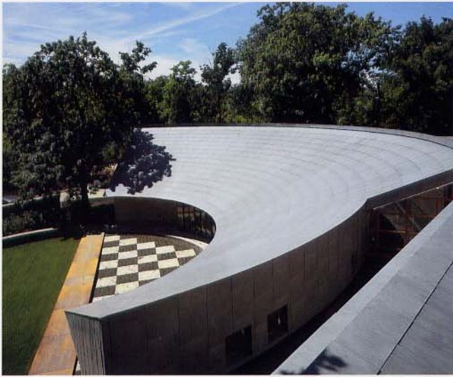
Kaplan residence, Illinois, USA
