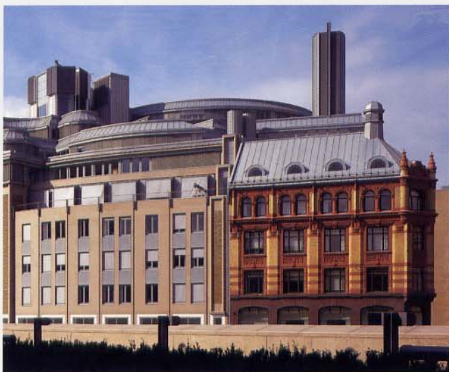
Government building R5, Oslo, Norway
